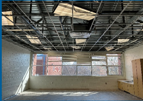
Ceiling Grids Install at Area B, C
