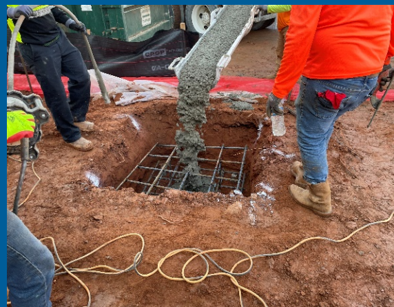
Metal Canopy footings being poured
