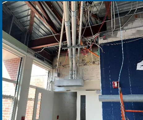
Main-Electrical Line Rough-in with pull can
